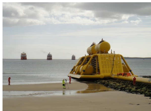
Figure 1-1: Launch of the template towhead. The bundle is seen on the shore side connected to the towhead.
