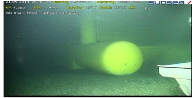
Figure 4-9: Picture taken four days after installation of FPSO towhead on rock berm.
