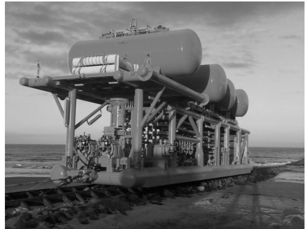
Figure 2-1: Picture of Knarr FPSO towhead during launch. The bundle is seen entering the water.
