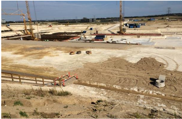
Figure 2: Excavation for basement level K2.
