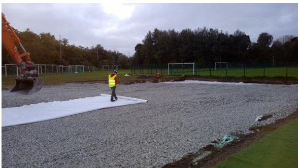
Figure 3. Foamed glass being spread on a sports area worksite (Foamit 2012).
