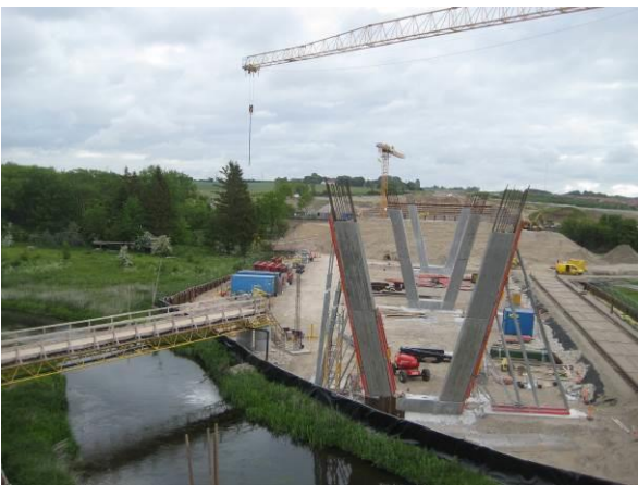
Figure 8: Construction of the bridge – overview of the site
