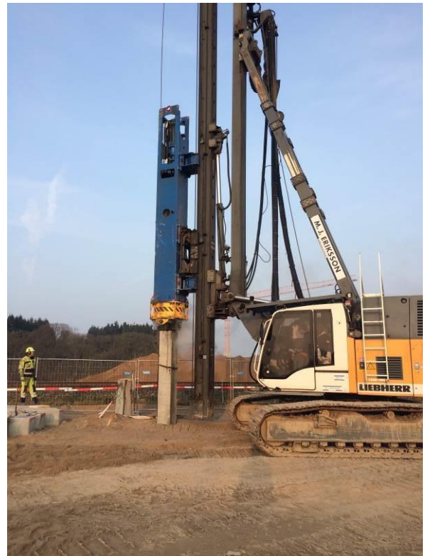
Figure 5: Construction of the bridge – installation of piles
