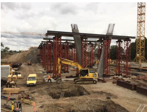
Figure 4: Construction of the bridge – excavation for temporary foundations for scaffolding
