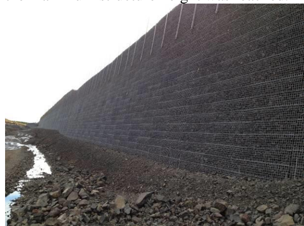
Figure 11 The completed structure.
