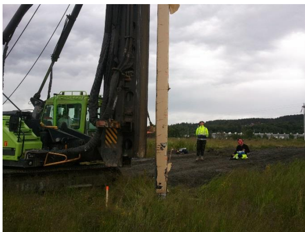
Figure 7: Test piling with PDA-testing
