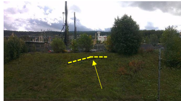
Figure 11: Surface crack in slope (marked with yellow dashed line)
