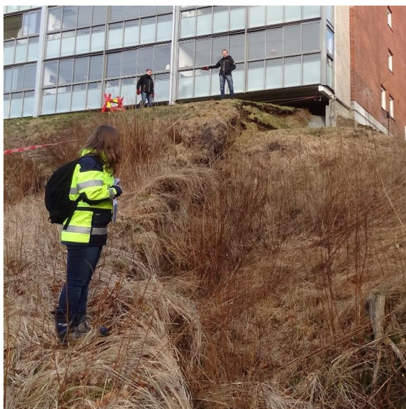
Figure 2 The backscarp of the slide. Vertical deformation 0,5-1 m.
