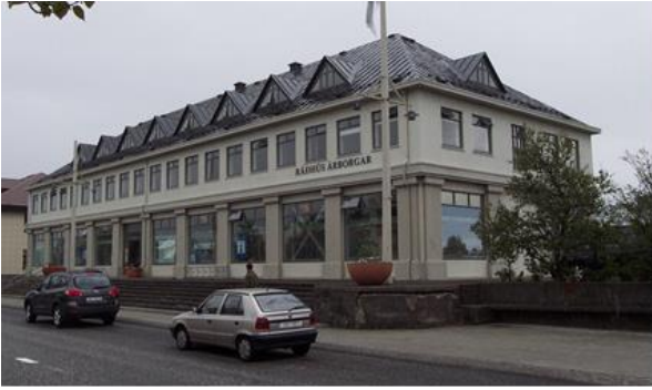
Figure 3 The Town Hall at Selfoss, view from NE.
