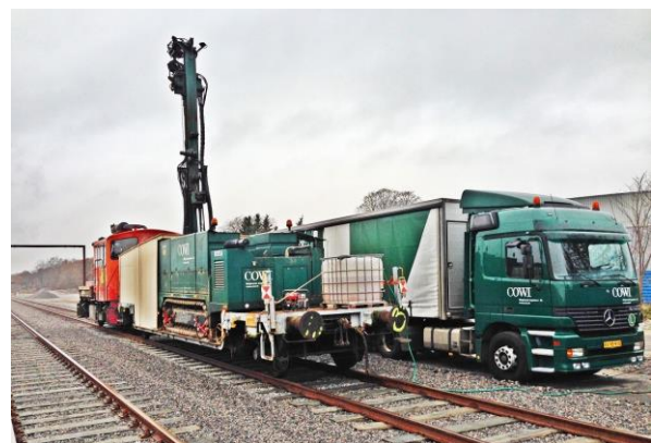
Figure 2, Drilling rig mounted on wagon ready for on-track work
